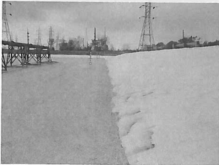
Warning layer along north slope (looking west).
