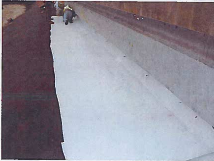
Looking south placing liner at weir.
