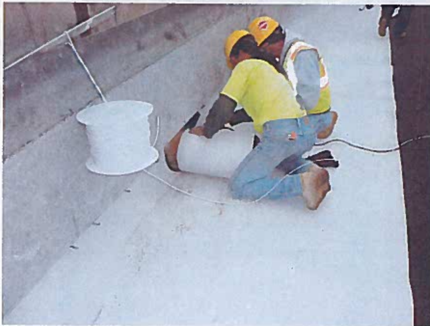
Looking north, working on placement of pipe collar around metal pipe.
