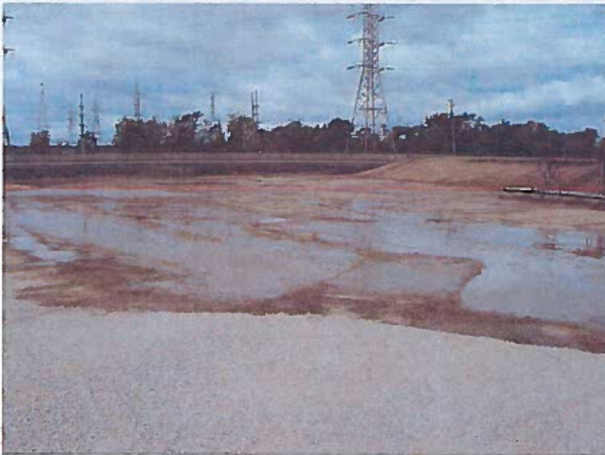
Looking northwest from top of ramp at pond subgrade.
