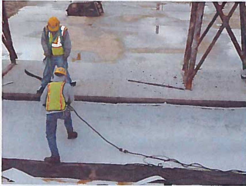
Welding liner to replaced welding strip (looking south).
