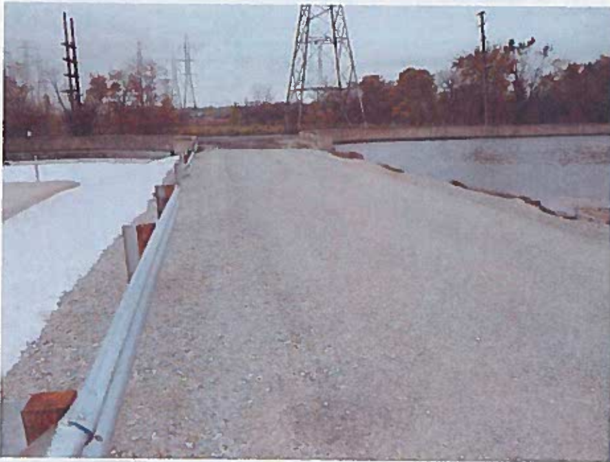
Guard rail between ash pond 2 and 3 (looking west).
