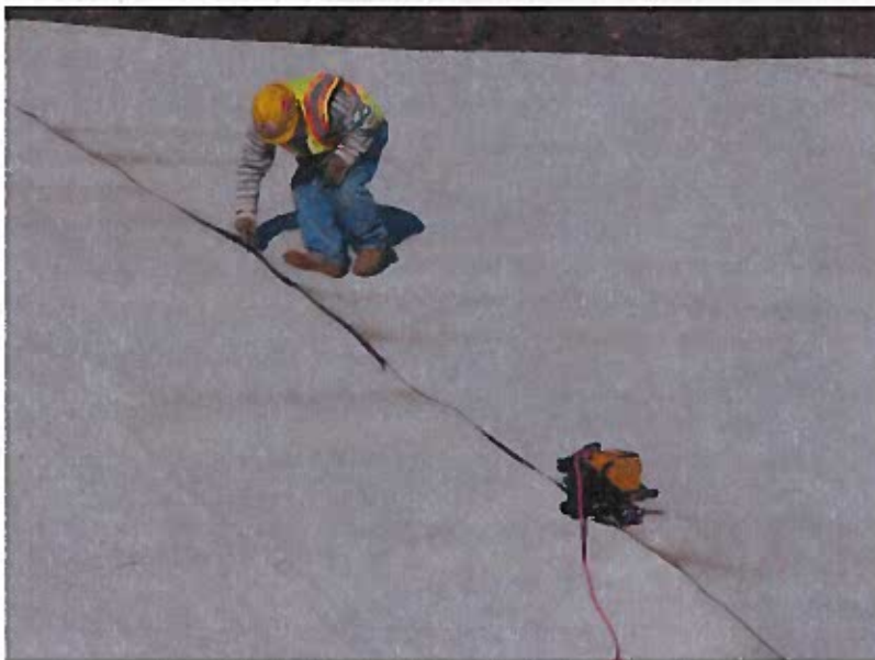
Thermal fusion welding apparatus
