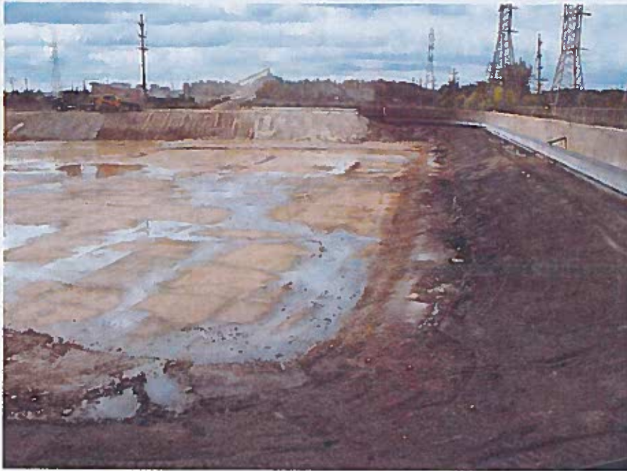
Looking south along the weir at subgrade.
