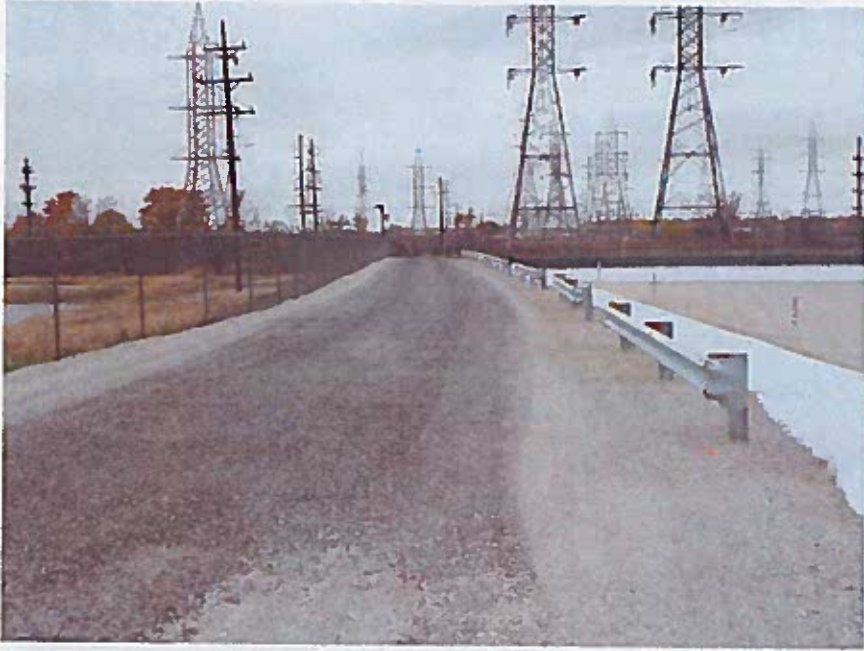
Guard rails placed along south slope (looking west).
